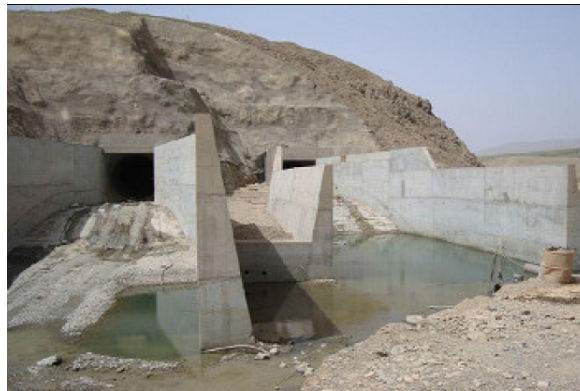
Figure 20. The outlet of diversion dam
