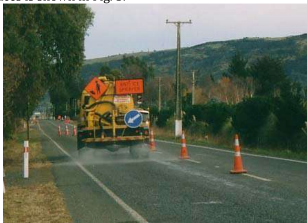
Fig 3. use of CMA in de-icing road surfaces in fluid state
