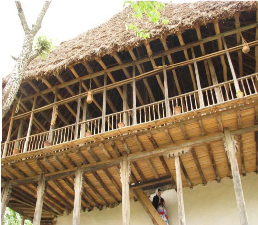
Figure 7. Traditional architecture of rural houses of Langroud city.
