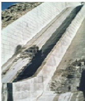
Figure1. Damage of cavitation-Karoon1 Dam
