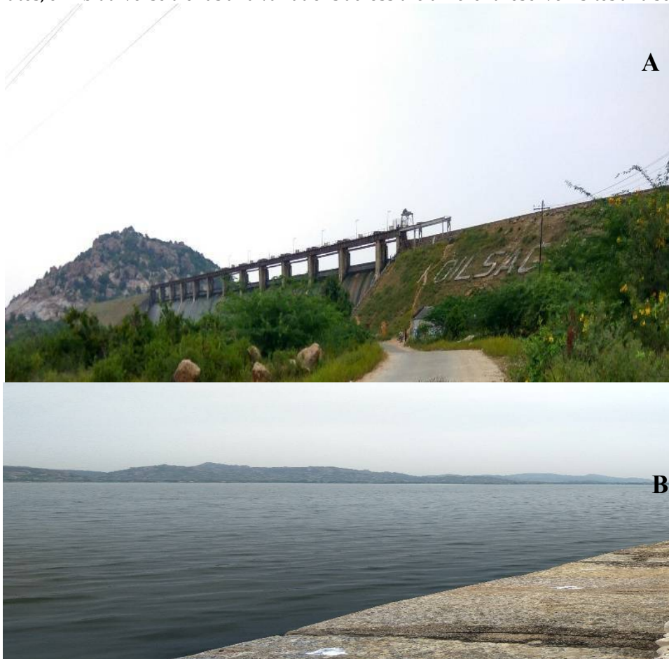
Figure 1: Koilsagar reservoir, (A) front view (B) back view
