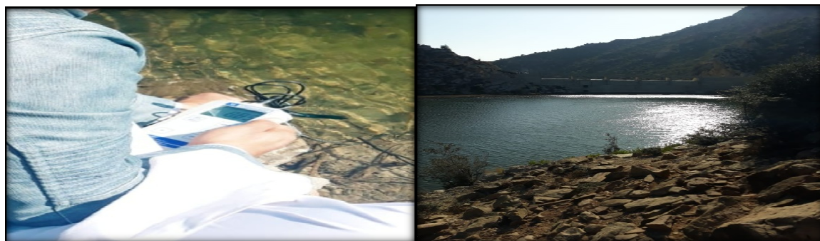
Fig 2: Site view of Mardankhel dam.
