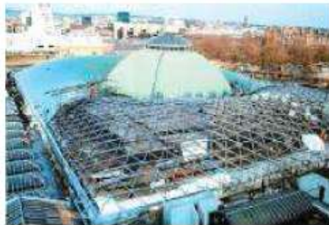
Figure 11. Great Court Roof of The British Museum during construction
