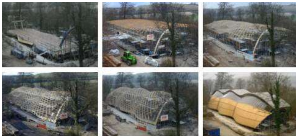
Figure (10) the construction of weald and downland open air museum, all figures [15].
