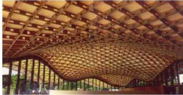
Figure 2. The use of continuous covering layer to create shell behavior [5]
