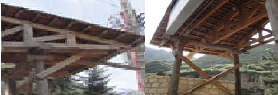
Picture 3- linking beams to columns with vernacular materials
