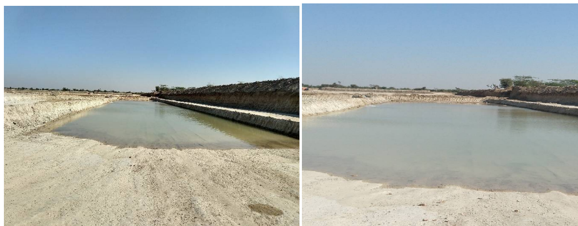
Figure 2. Rain water storage system in Giral mines, Barmer
